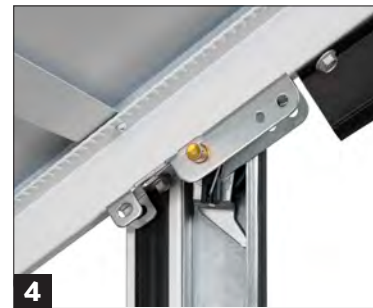
Guide rail & anti-drop safety mechanism
